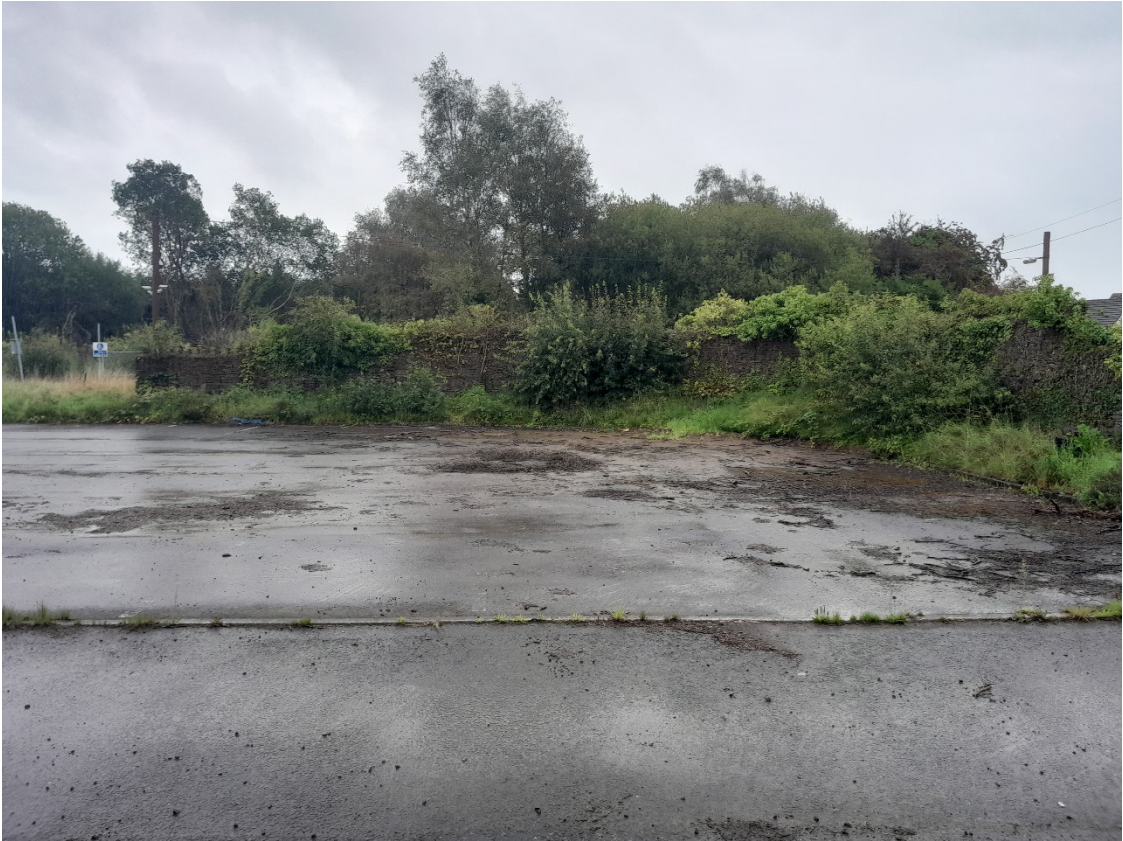
Image EDP A1.21: East facing view of the identified c. 1901 east stone boundary wall to the former Glamorgan Works ( GGAT01225w ).
