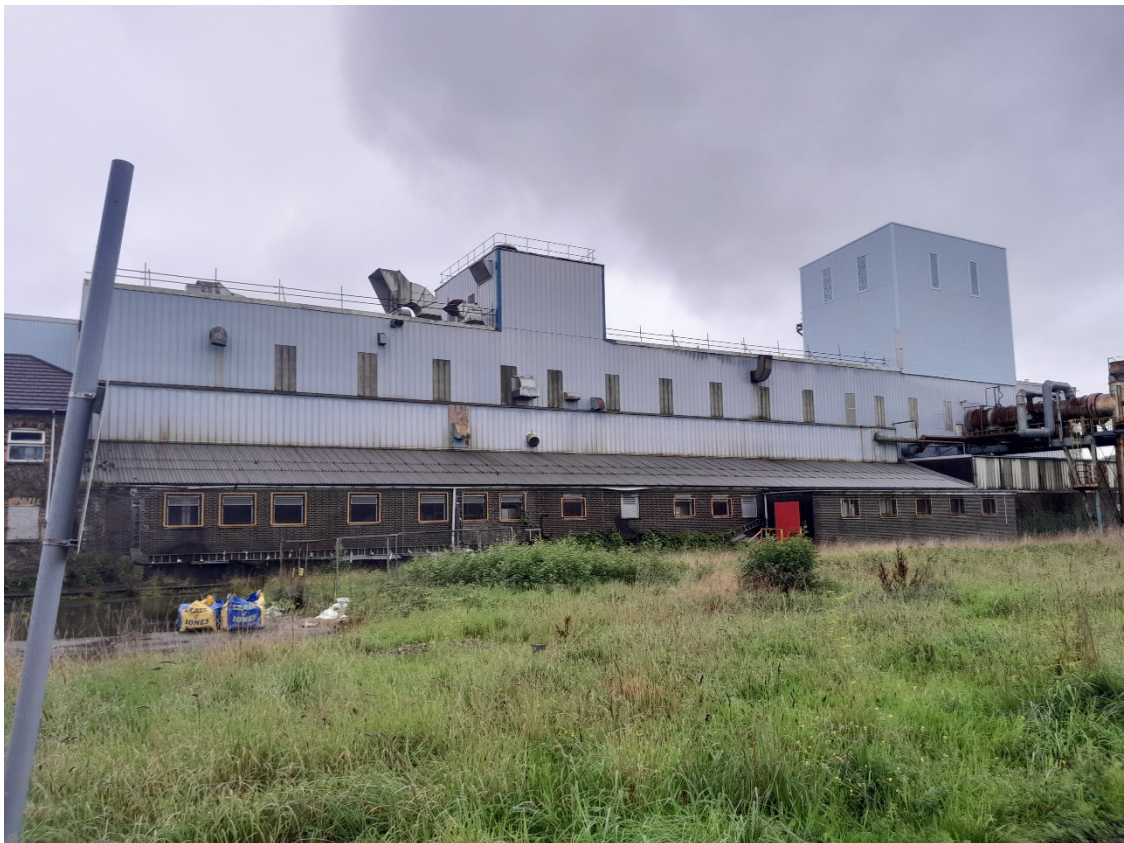
Image EDP A1.9: North-west facing view of the building complex within the Site from its east side.
