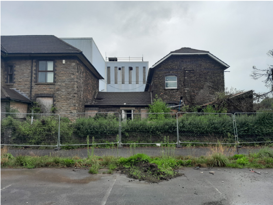
Image EDP A1.2: North facing view of the extant historic connecting 'L-shaped' stone-built buildings associated with the former Glamorgan Works ( GGAT01225w ) within the Site. Twentieth century renovation and alteration is visible including the modern roof, wooden and white PVC window casements and altered doorways.
