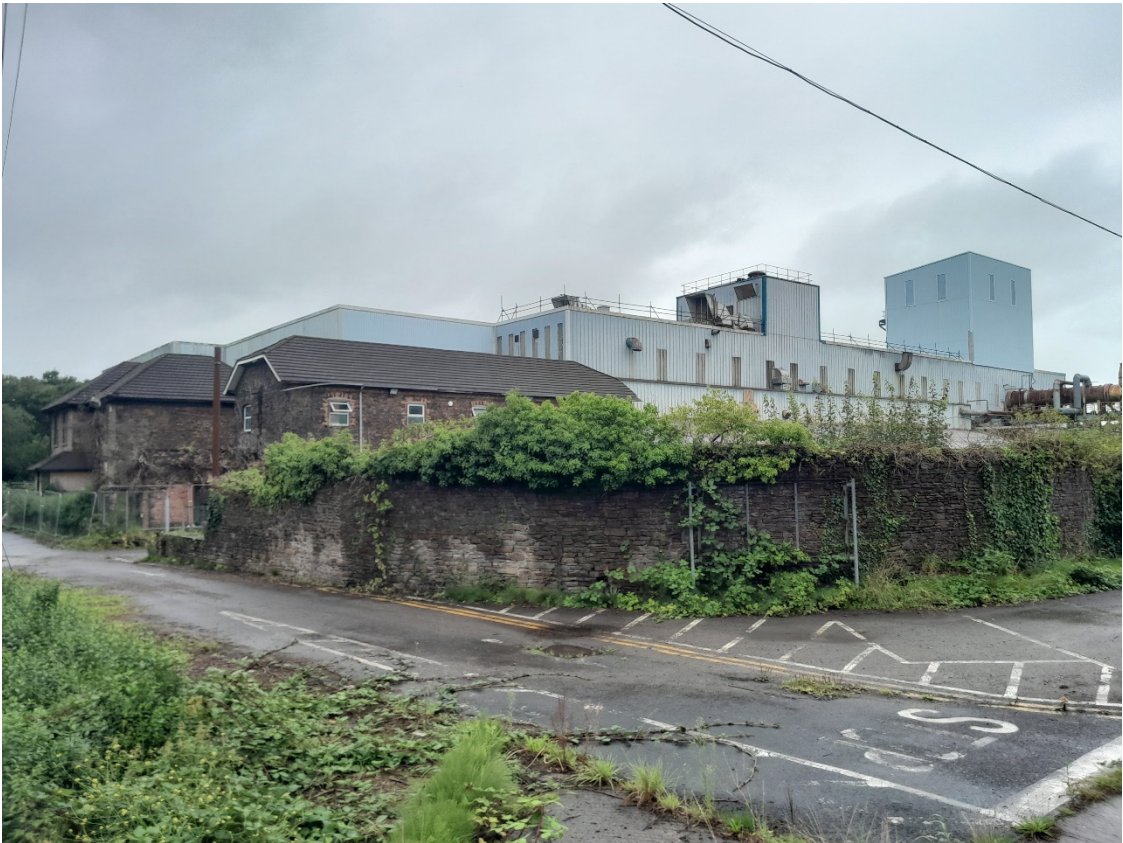
Image EDP A1.20: North-west facing view of the identified c. 1901 east stone boundary wall to the former Glamorgan Works ( GGAT01225w ).
