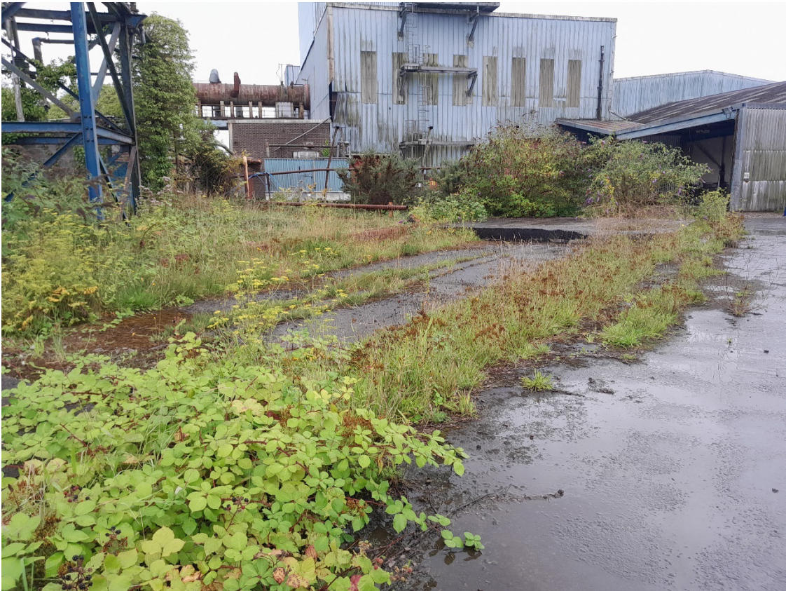
Image EDP A1.16: South facing view of tank platforms to the north of the Site's building complex.
