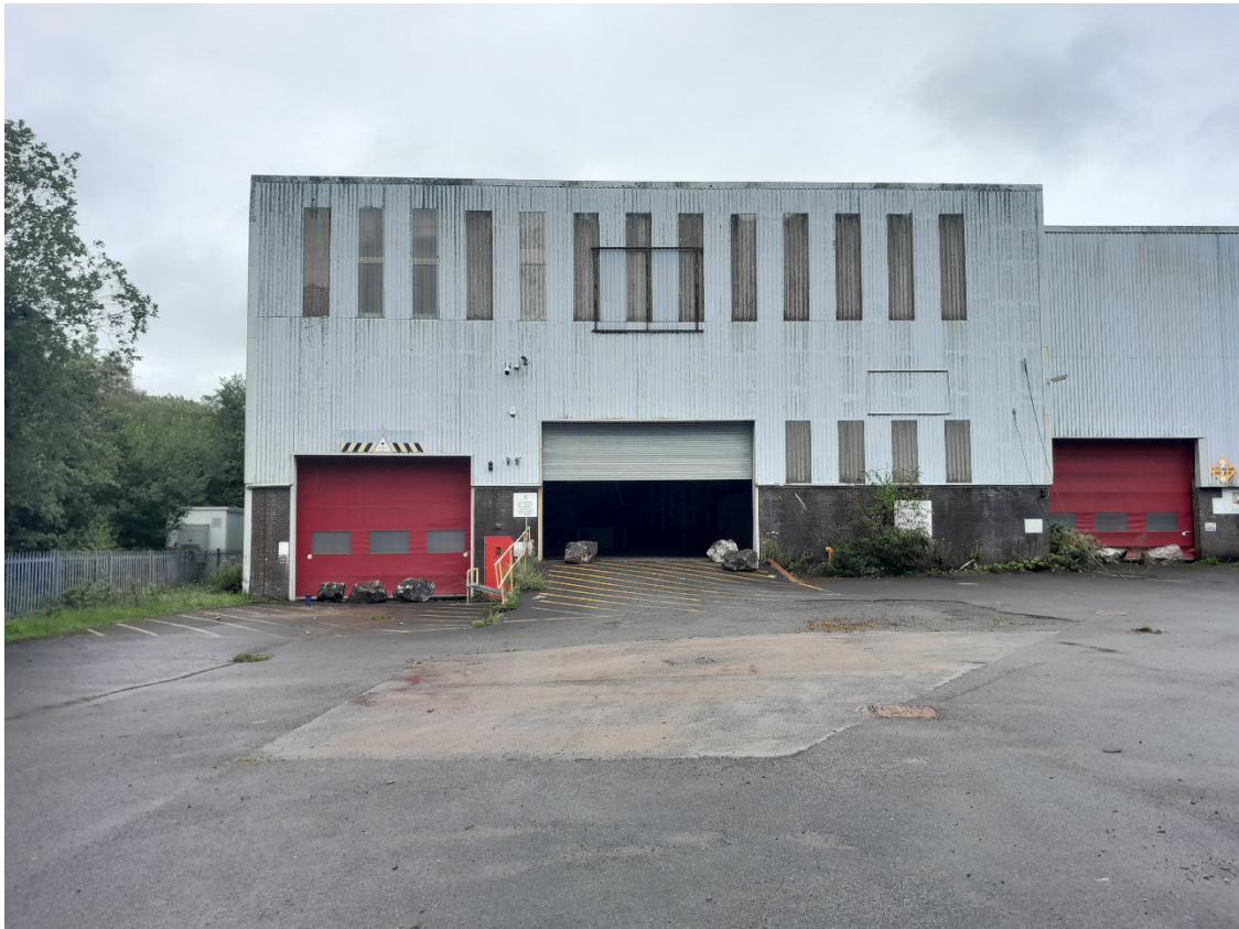
Image EDP A1.8: North facing view of the building complex within the Site from its south-west end.
