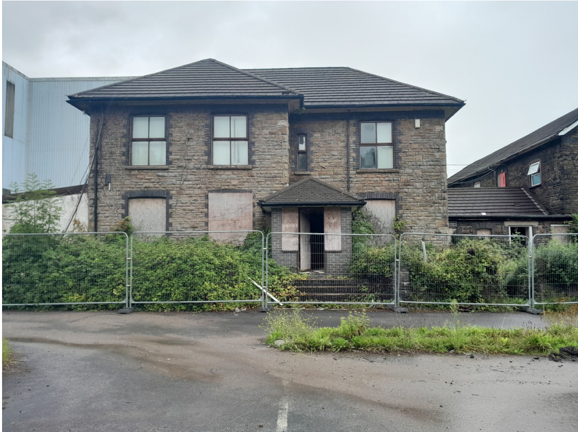
Image EDP A1.1: North facing view of the extant historic connecting 'L-shaped' stone-built buildings associated with the former Glamorgan Works ( GGAT01225w ) within the Site. Twentieth century renovation and alteration is visible including the modern roof, brick porchway extension, wooden window casements and adjoining lean-to extension on the west side of the building.
