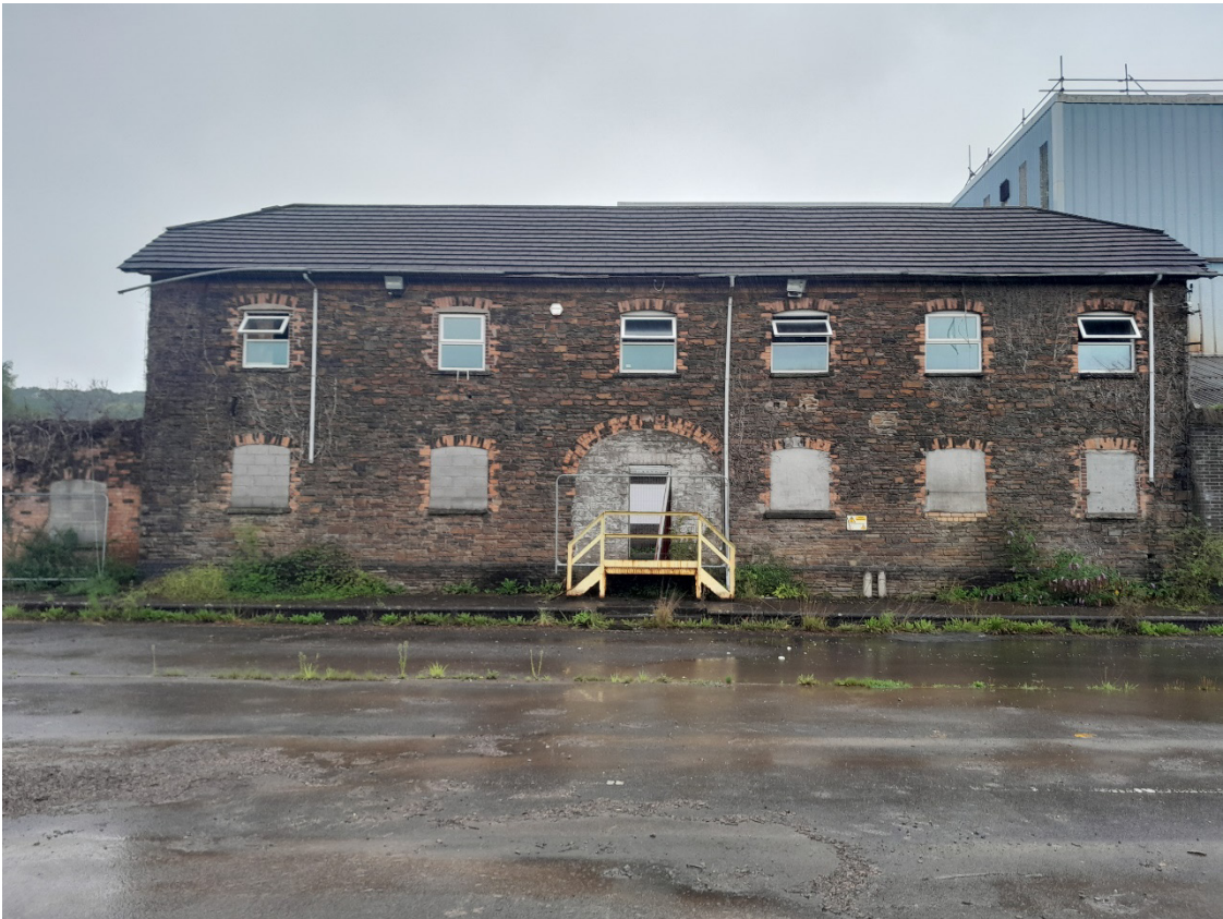
Image EDP A1.4: West facing view of the extant historic connecting 'L-shaped' stone-built buildings associated with the former Glamorgan Works ( GGAT01225w ) within the Site. Twentieth century renovation and alteration is visible including the modern roof, white PVC window casements, altered doorway and red brick building extension on the south side of the building.
