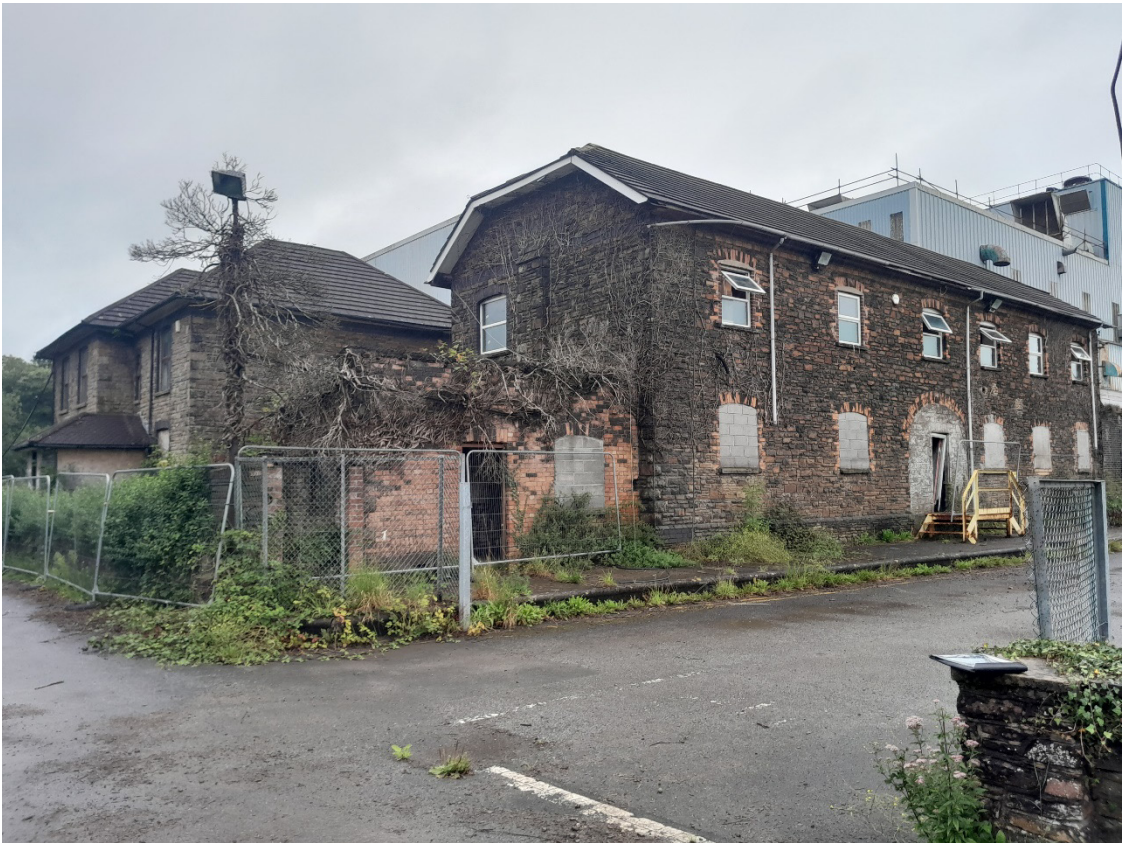
Image EDP A1.3: North-west facing view of the extant historic connecting 'L-shaped' stone-built buildings associated with the former Glamorgan Works ( GGAT01225w ) within the Site. Twentieth century renovation and alteration is visible including the modern roof, white PVC window casements, altered doorway and red brick building extension.
