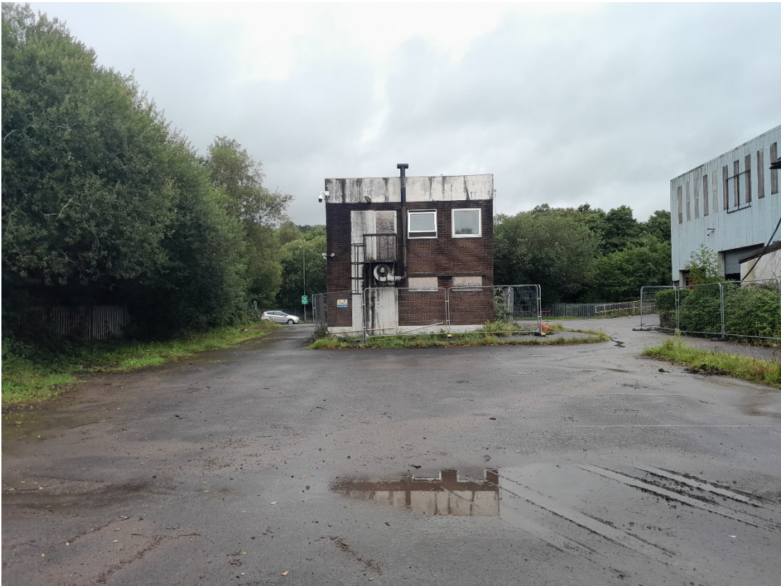
Image EDP A1.13: West facing view of extant outbuilding to the south of the main building complex within the Site. The brown brick and flat roof structure most likely dates between 1972-1992, alongside the majority of the extant building complex within the Site.
