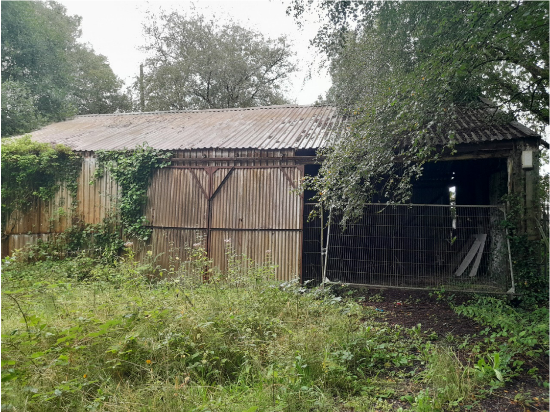
Image EDP A1.7: South facing view of the identified 1960s-1970s corrugated steel shed (2/2) within the south end of the Site.
