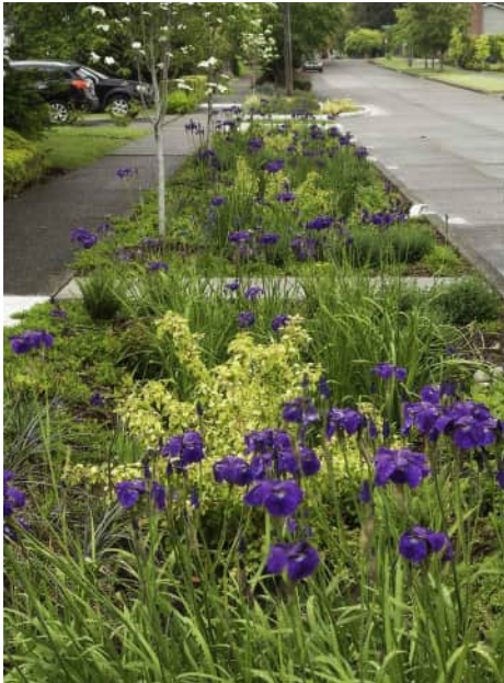
Rain gardens through the site, managing surface water and enlivening the street.
